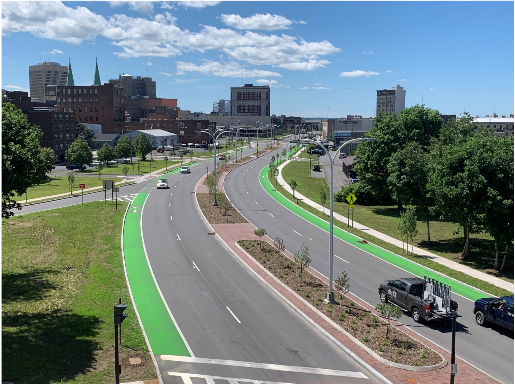
Completed Project – Route 55 Looking West Between 2 nd Street and John Street
