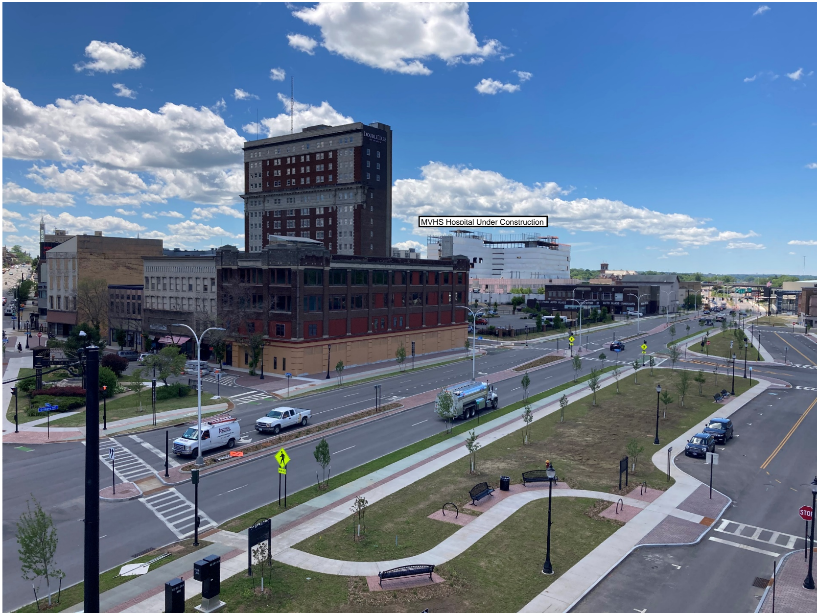
Completed Project – Route 5S Looking West From Genesee Street
